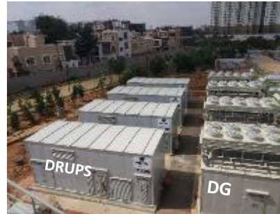
India's first Medium voltage Isolated parallel bus DRUPS system
